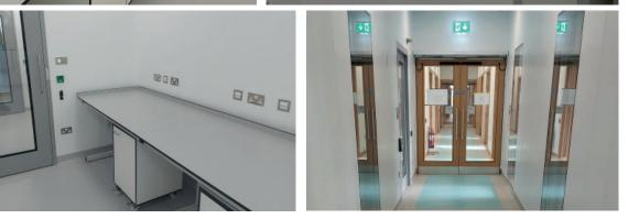
"The MIDDAS M100 wall system was selected to deliver on the facilities stringent requirements in terms of airtightness, cleanability, surface finish, robustness, acoustics, and integration of services."
