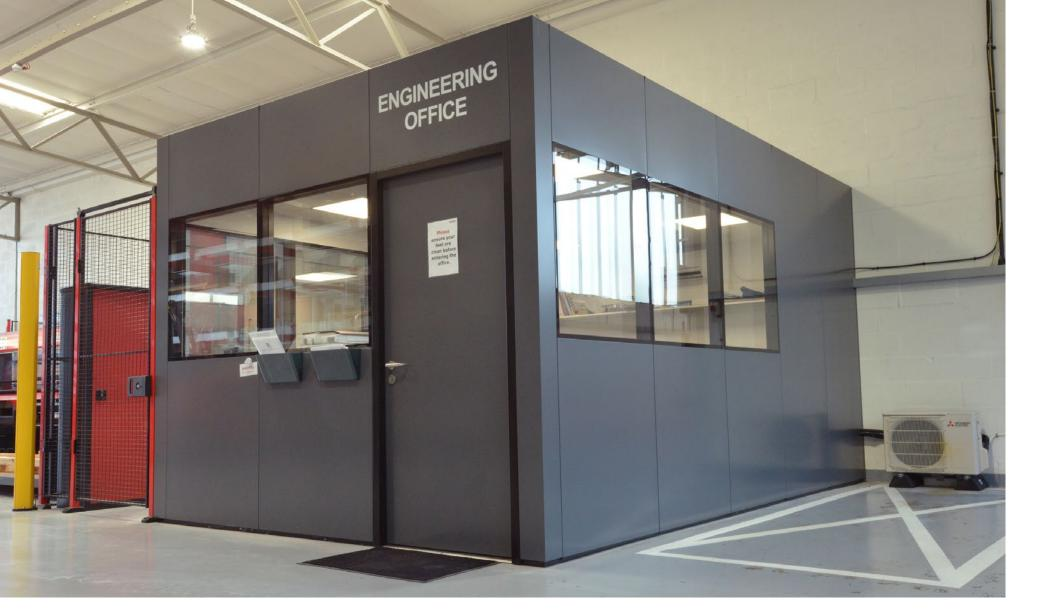
MIDDAS Freestanding Structures can be constructed within any existing building, including storage warehouses, manufacturing facilities and distribution centres, to create an envelope that is entirely independent of the building structure. Our structures are built to support the full load of distributed M&E services from the building slab, not the framework, at a force up to 2.5kN/m2 plus the weight of the ceiling.
